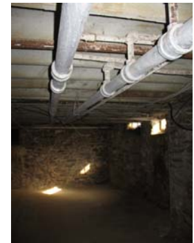
"Insulating heating pipes in unoccupied spaces"
